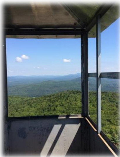
St. Regis Mountain Fire Tower
