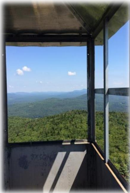
St. Regis Mountain Fire Tower
