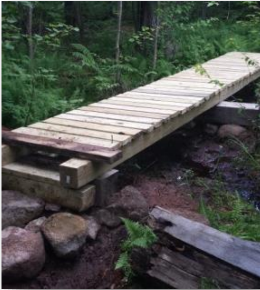
Footbridges built by stewards at Wanakena.
