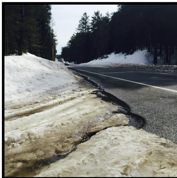
Image 9. Direct road salt runoff coming off of NYS RT 30 during a thawing event in the spring of 2015. The chloride concentration of this melt water was approaching 5,000 mg/L which is ¼ the concentration of sea water.
